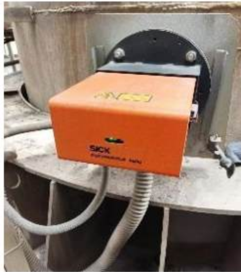
Sick Opacity meter in all stacks
